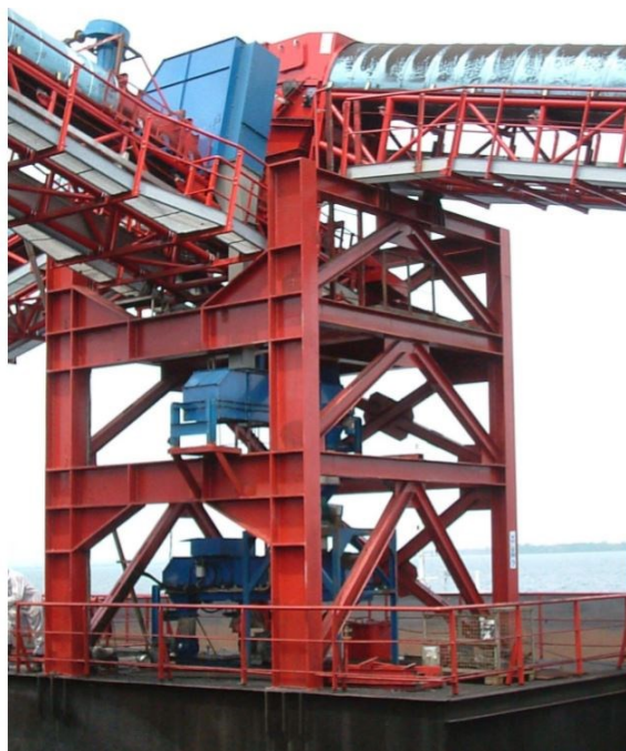
Fig. 6 The sampling system from the conveyor belt located near the dumping
