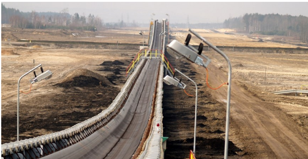
Fig. 1 Overland belt conveyor
