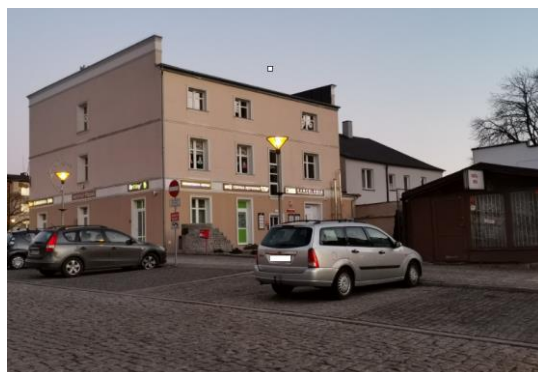
Fig. 2 Cars parked perpendicular to the traffic lane
