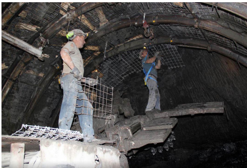
Fig. 1 Mounting of a steel arch support using a roadheader
