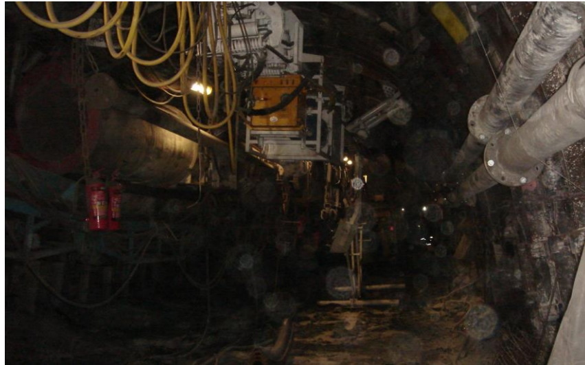
Fig. 9 The modular installation and transport assembly installed in an underground excavation
